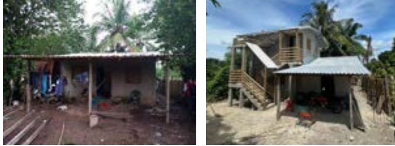
Before (left) and after (right) Build Change and Honduran Red Cross technical and financial support for retrofit and expansion of Irma Mercedes Mardiaga’s home
