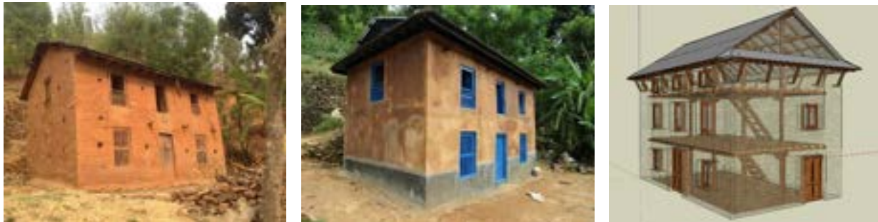
Caption: A typical stone masonry in mud mortar house in Eklephat village in Nepal before (left) and after (center) being retrofitted. (Right) 3D structural model of a typical stone masonry house in rural Nepal.
