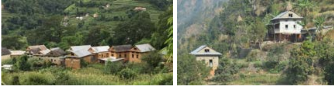
Caption: Stone masonry houses are similar in size and configuration and the most common typology in rural Nepal
